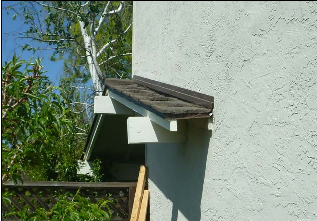
Reverse Sloped Flashing
